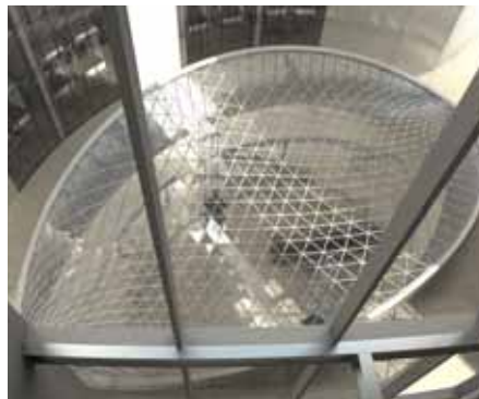
Figure 6c. View to Skybridge dome from glass elevator
