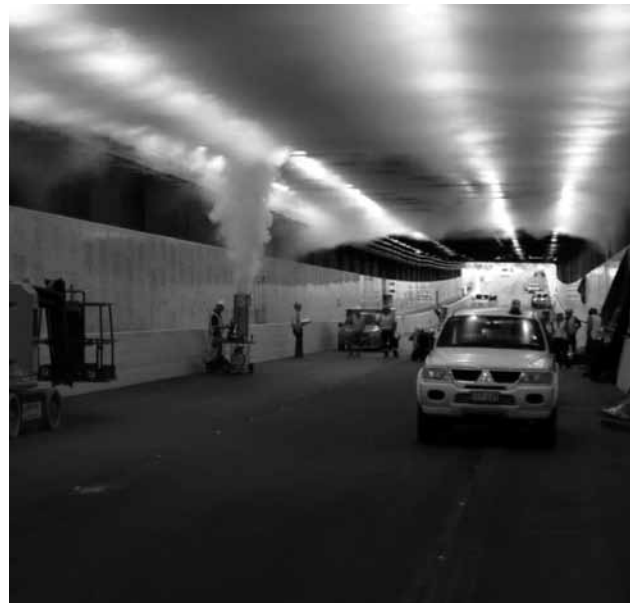
Smoke testing in the Tugun Bypass Tunnel, March 2008.
